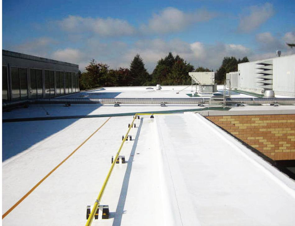
effective solution: they jacked up the air handlers just enough to remove the sleeper covers and old roofing system and install the vapor barrier and insulation; and then they took one 10-foot-wide sheet of the Sika Sarnafil membrane and slid it up and over the sleepers at each of the air handlers. This way the edges of the sheets could be welded to the outside edges, eliminating any welding underneath the air handlers.
